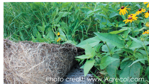
A native vegetated mat being rolled out.
